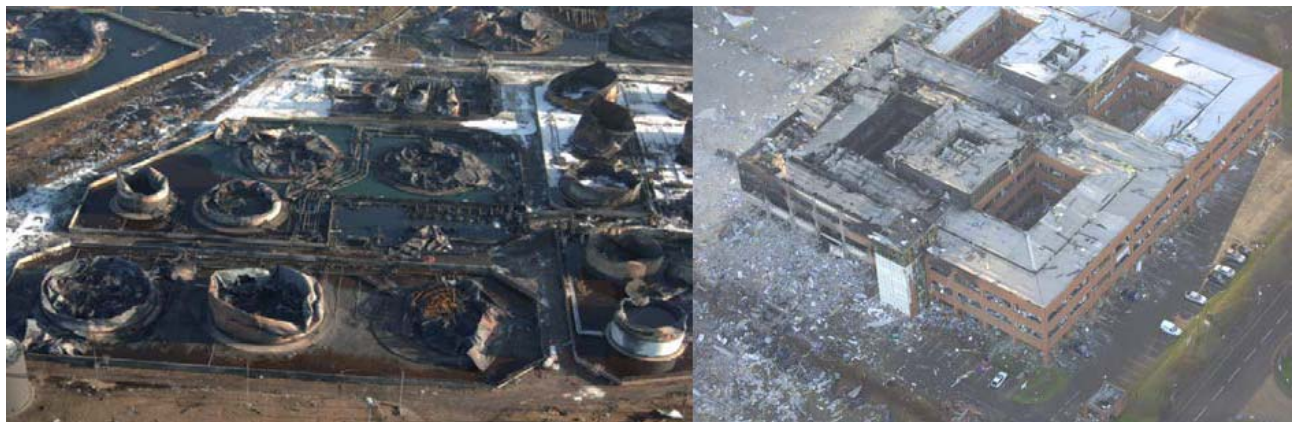
Figure 1-1. Oil terminal just outside London in Buncefield, U.K. A tank overfill resulted in vapor cloud explosion and formation of the largest smoke cloud in western Europe since WW II. Fortunately there were no fatalities (1)
