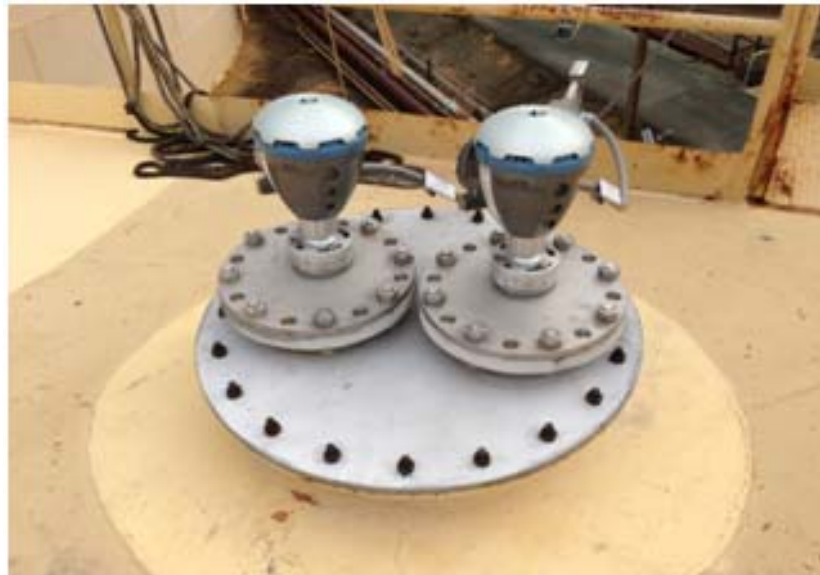
Figure 1-5. The industry trend is to use two continuous sensors for both level and overfill prevention measurements, here exemplified with Rosemount 5900 Radar Level Gauges
