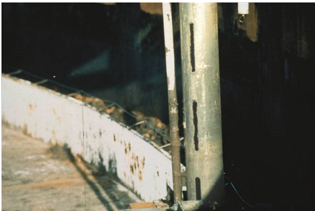
Figure 12: The Low Loss Mode Enables Full Accuracy also in Old and Worn Still-Pipes
