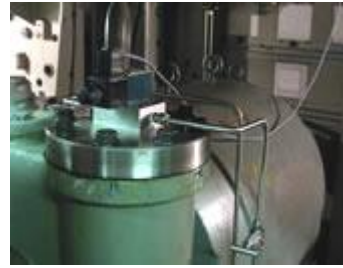
Figure 8. Large XX Flange – After
