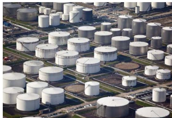
Smart wireless enables overfill protection of crude oil storage tanks during off loading from ships
