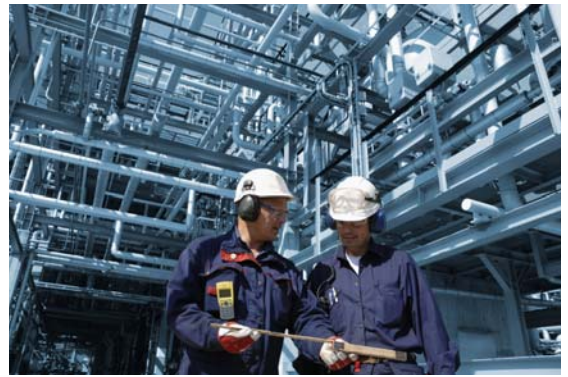
Dense piping, vessels, and tanks are a challenge to wiring, and to non-mesh wireless technologies
