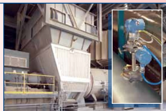
Rosemount 3095MFA Mass Probar Flowmeter
