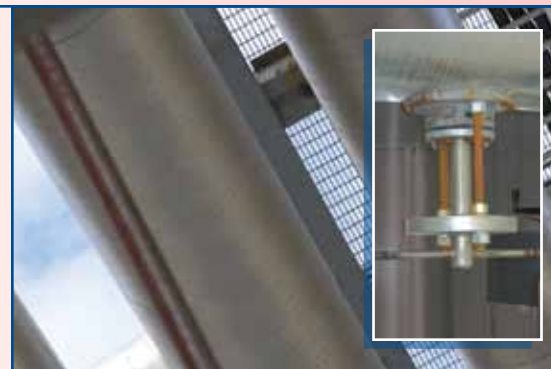
Rosemount 3051SFA Probar® Flowmeter
