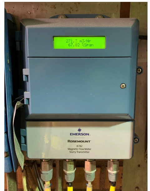
Rosemount 8782 Transmitter for Slurry Applications
