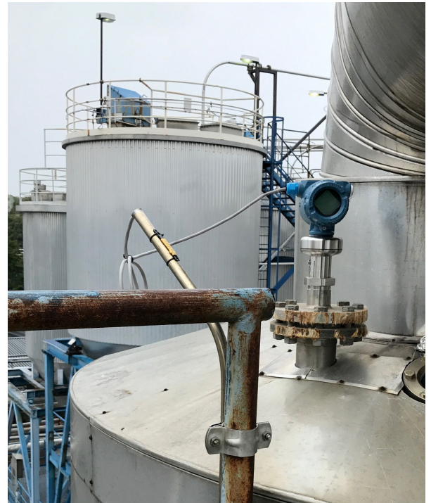
Illustration shows the Rosemount 5408 installed on a cyclone reactor.
