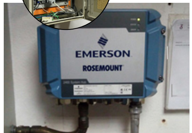
After: Newly installed Rosemount 2460
