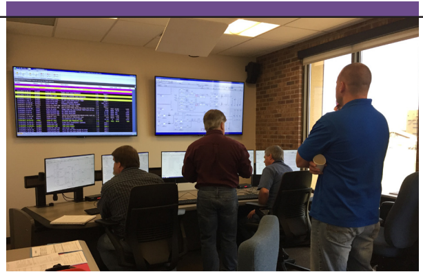
Emerson's high-fidelity Ovation digital twin simulator is in use now for training, control logic testing, patch verification and continuous improvement of plant operating procedures at Rawhide Energy Station.
