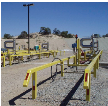
SWD offloading site
