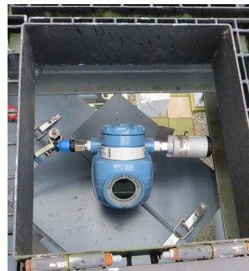
To enable use of the diagnostics, a SmartWireless THUM Adapter was added to each Rosemount 5300.
