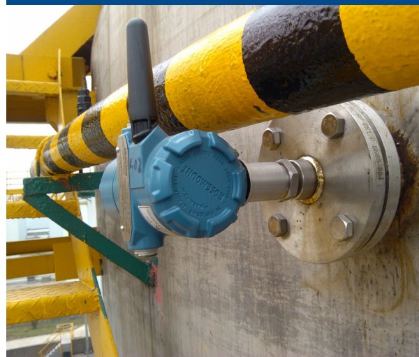
Side-mounted Rosemount 2160 Wireless Vibrating Fork Level Switch
