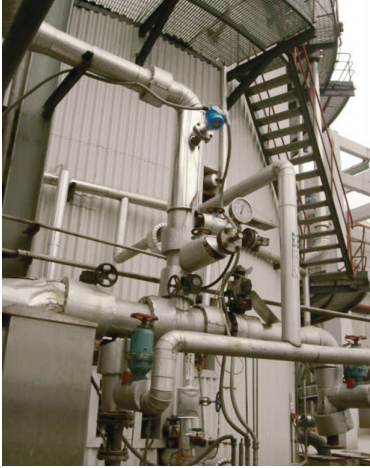
Installation of a Micro Motion Fork Density Meter in FGD process pipeline
