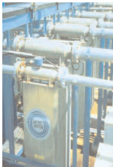
Jetty for oil tank storage.
