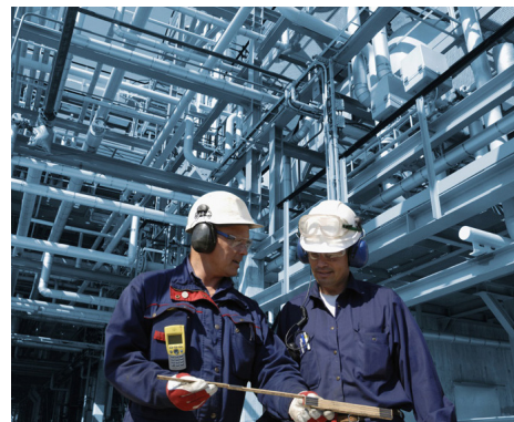
Dense piping, vessels, and tanks are a challenge to wiring, and to non-mesh wireless technologies
