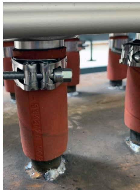
Connection to the boiler's orifices at the bottom of the ASCO Series 355 tanks with ASCO Series 353 valves
