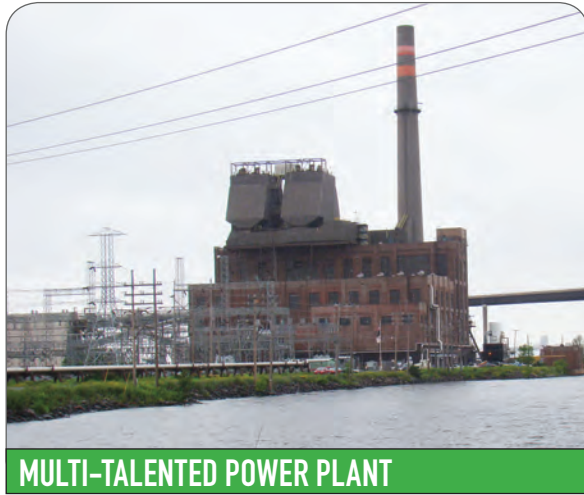
Figure 1: The M.L. Hibbard Renewable Energy Center power plant in Duluth, Minnesota has a multi-fuel, traveling-grate boiler that burns both wood waste and coal. The problem was that it operated almost all the time on manual controls.
