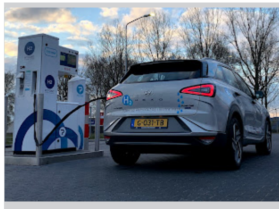
Dispenser with installed Emerson`s Micro Motion HPC015 Coriolis flow meter that fills vehicles with hydrogen under high pressure
